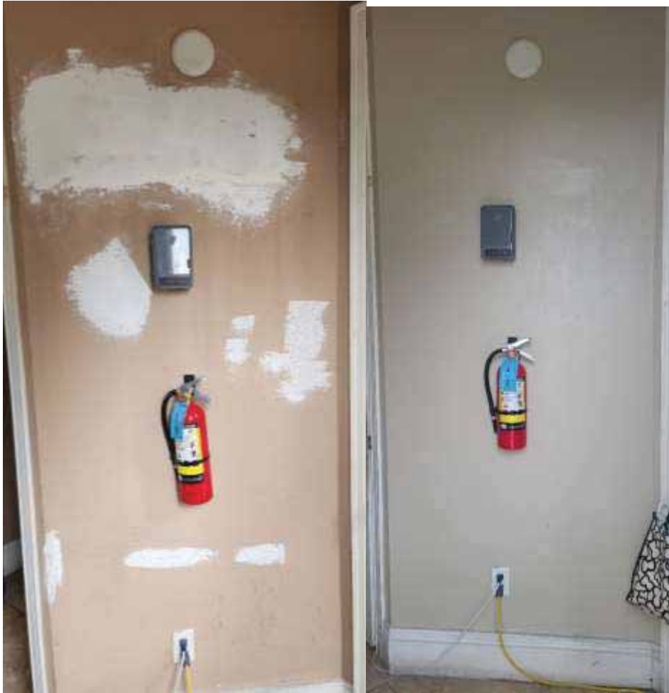
GUARD HOUSE PAINTING BEFORE & AFTER
