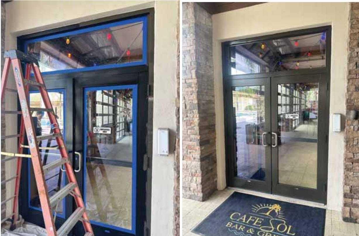
Cafe Door Before and After
